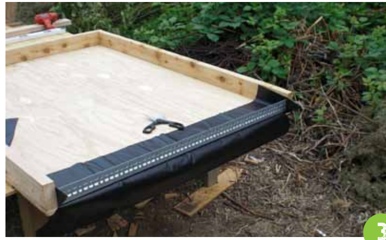
USE REDUNDANT SYSTEMS FOR WATERPROOFING
