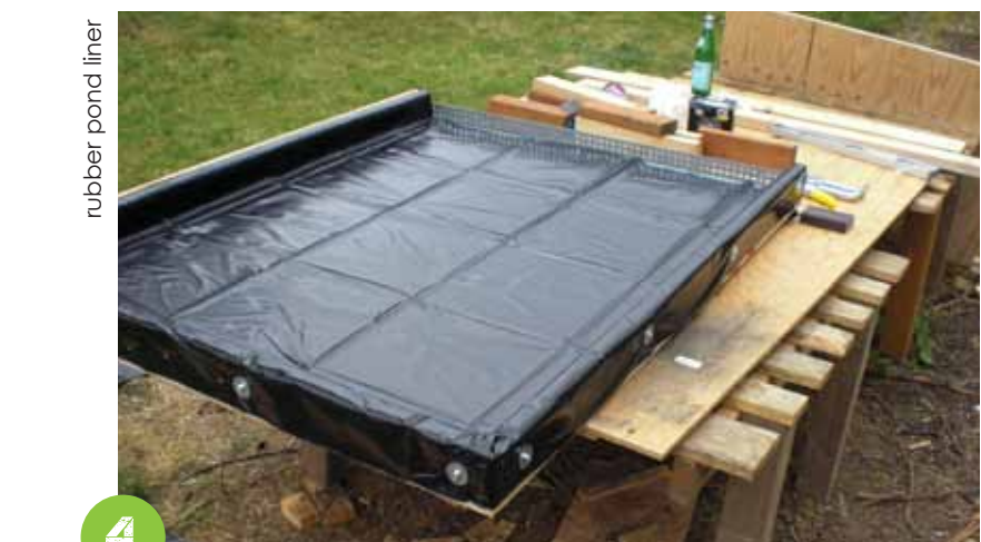
PROVIDE A CONTINUOUS WATER-TIGHT MEMBRANE
