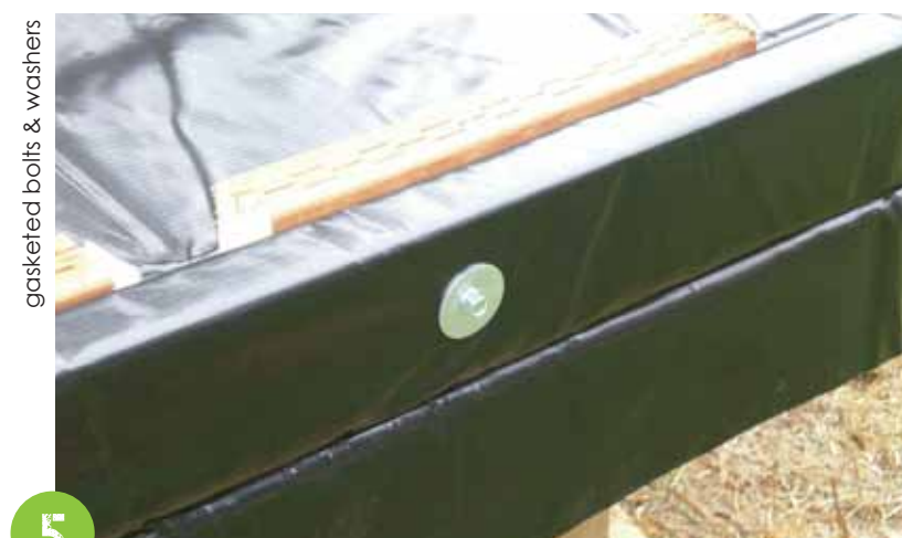
ATTACH FASTENERS ON EXTERIOR TO MAINTAIN ROOF
