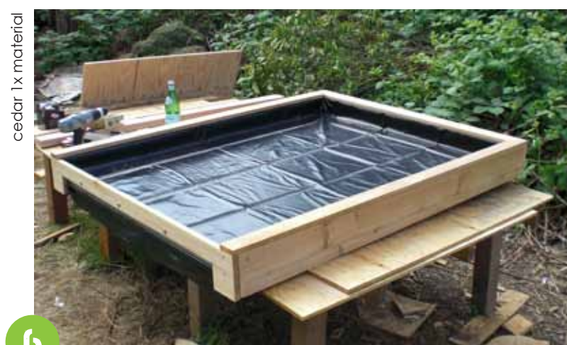
PROTECT AND CONCEAL WITH EXTERIOR CLADDING
